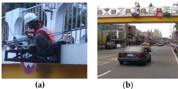
Fig.5. System installation, (a) system under construction, (b) system after construction.
