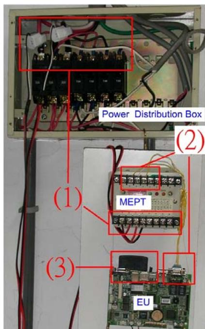
Fig. 10. Photo showing the deployed EU and MEPT for monitoring the power consumption of a power distribution box.
